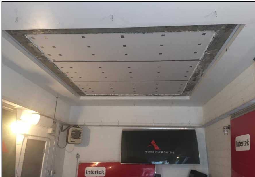
Receive Room View of Test Specimen Installation
