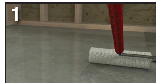
1 Roll on Protecto Wrap #6000 Primer, allow 20-30 minutes to dry.
