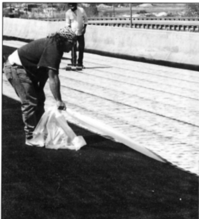
Release film removes easily after positioning membrane on overlap.
