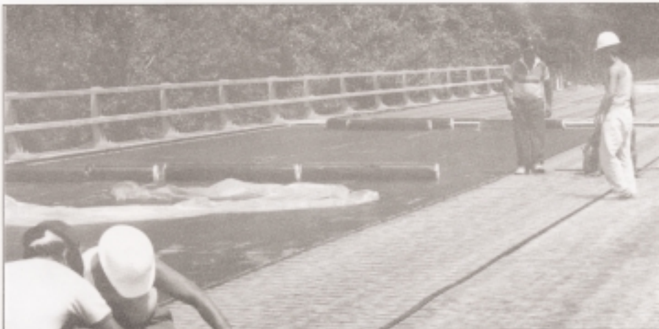
Silicone coated release film on the bottom of M-140A(R) and M-400A(R) allows the membrane to be easily positioned on the deck.
