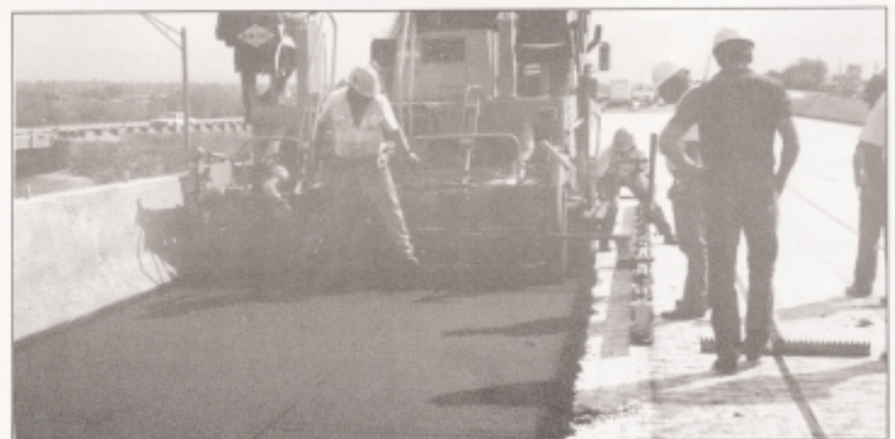
Overlay can be placed immediately after membrane installation.
