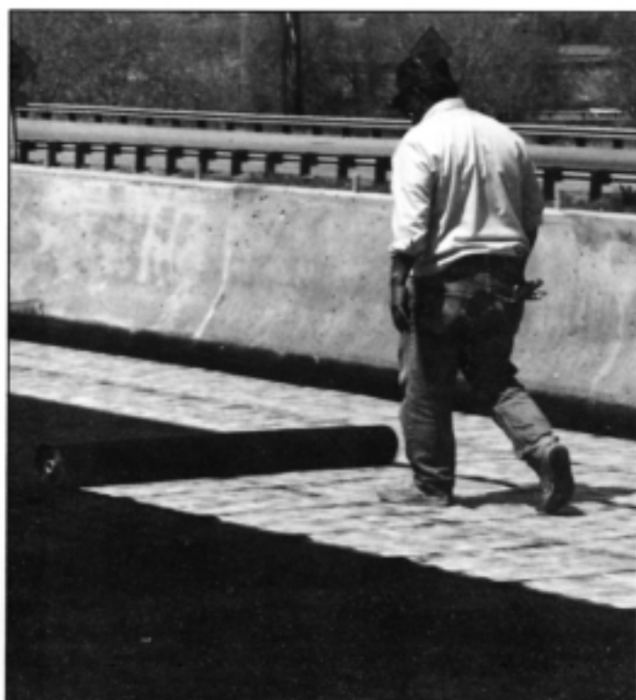
M-140A(R) AND M-400A(R) kick out for ease of positioning and instalment.
