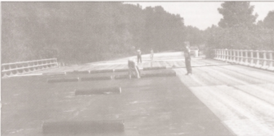
Staging roles of membrane increases production rates.
